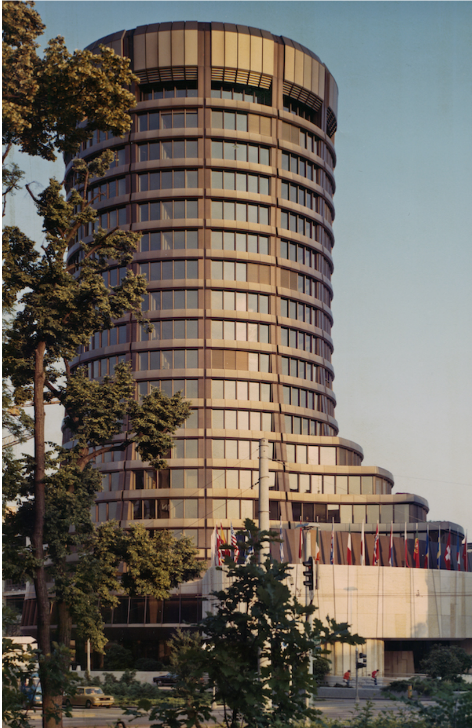
The BIS tower building in Basel, photographed 1978, a year after its completion. (BISA.7.27.1.BUI.2.Historical.photos.046)
